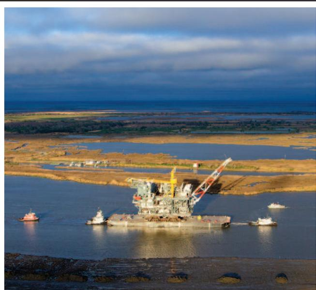
The 7,500-ton, three-level topsides departed Houma, La., in March 2014 in route to the Tubular Bells Field. The FPS was the first classic spar facility to be built entirely in the United States, with the topsides and hull fabrication work creating thousands of jobs in multiple states.
