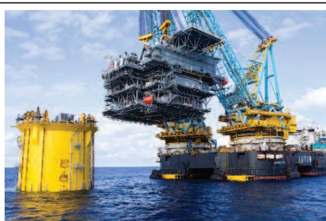
The Saipem 7000 heavy-lift vessel installs the topsides on the classic spar hull stationed in more than 4,000 feet of water. Production operations commenced within eight months of the date of this photo, completing a fast-track schedule that brought Tubular Bells from project sanctioning to first oil in the span of three years.
