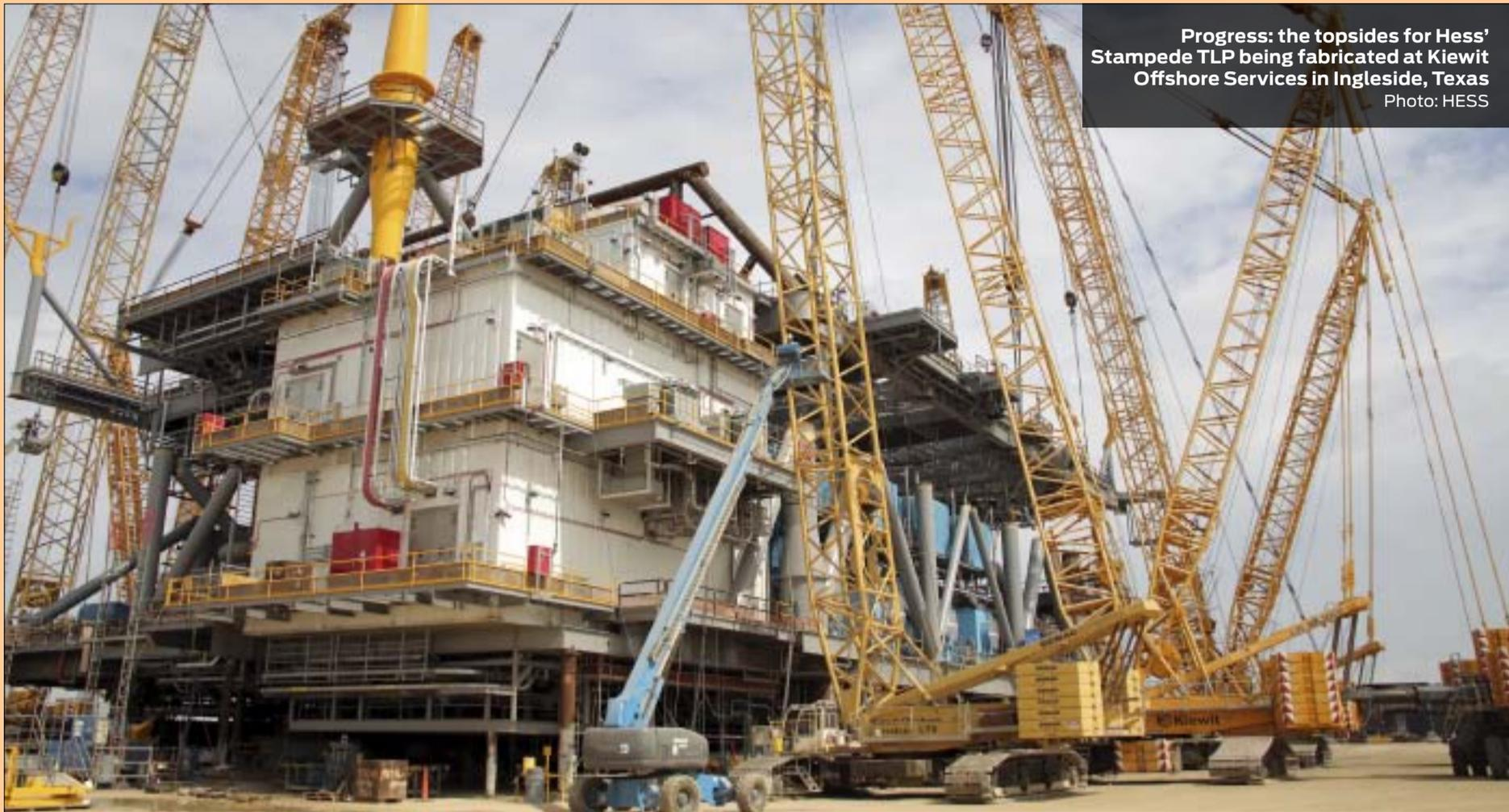
Progress: the topsides for Hess' Stampede TLP being fabricated at Kiewit Offshore Services in Ingleside, Texas
