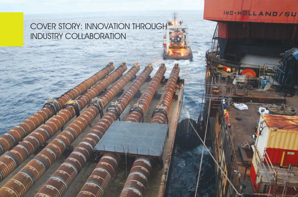
The 120-m-long anchor piles were loaded onto transport barges at Gulf Marine Fabricators. It took the barges three days to reach the Stampede Field from Ingleside, Texas. (Source: Hess Corp.)
