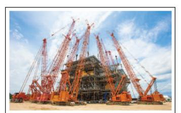
The topsides for the *Gulfstar One* FPS for the Tubular Bells Field were designed to process 60,000 barrels of oil and 135 MMcf of gas a day along with up to 60,000 bbl/d of water injection. Shown here is the main deck lift in May 2013 at Gulf Island Marine Fabricators' construction yard in Houma, La.
