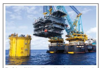
The Saipem 7000 heavy-lift vessel installs the topsides on the classic spar hull stationed in more than 4,000 feet of water. Production operations commenced within eight months of the date of this photo, completing a fast-track schedule that brought Tubular Bells from project sanctioning to first oil in the span of three years.
